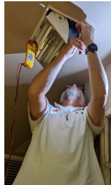
Mike King replacing light fixtures.
