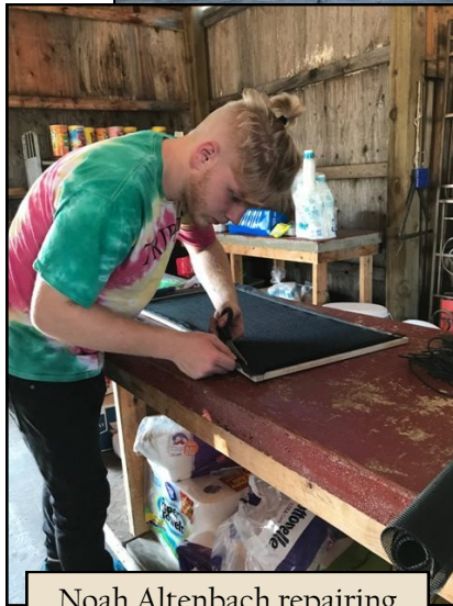
Noah Altenbach repairing a window screen
